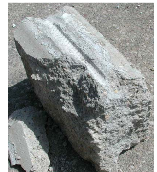
Figure 1: Sand Mix Grout in Panel
