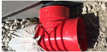
Connecting Wall Drain Pro To T-Drain
