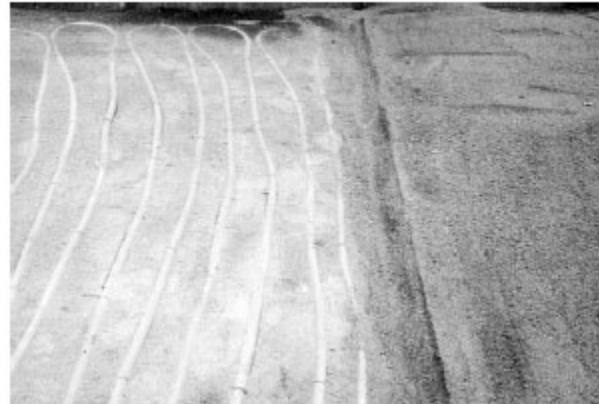
Figure 7. Screeding bedding sand must be done without moving or damaging pipes or wires for melting snow.
