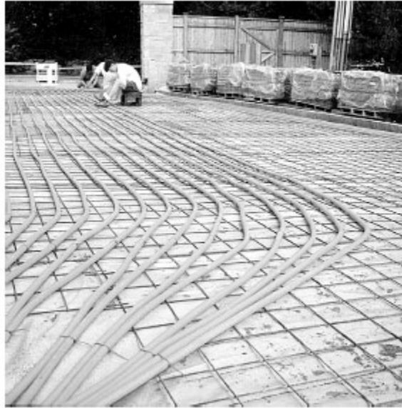
Figure 4. The heating system is tied to a wire mesh anchored into the compacted aggregate base.
