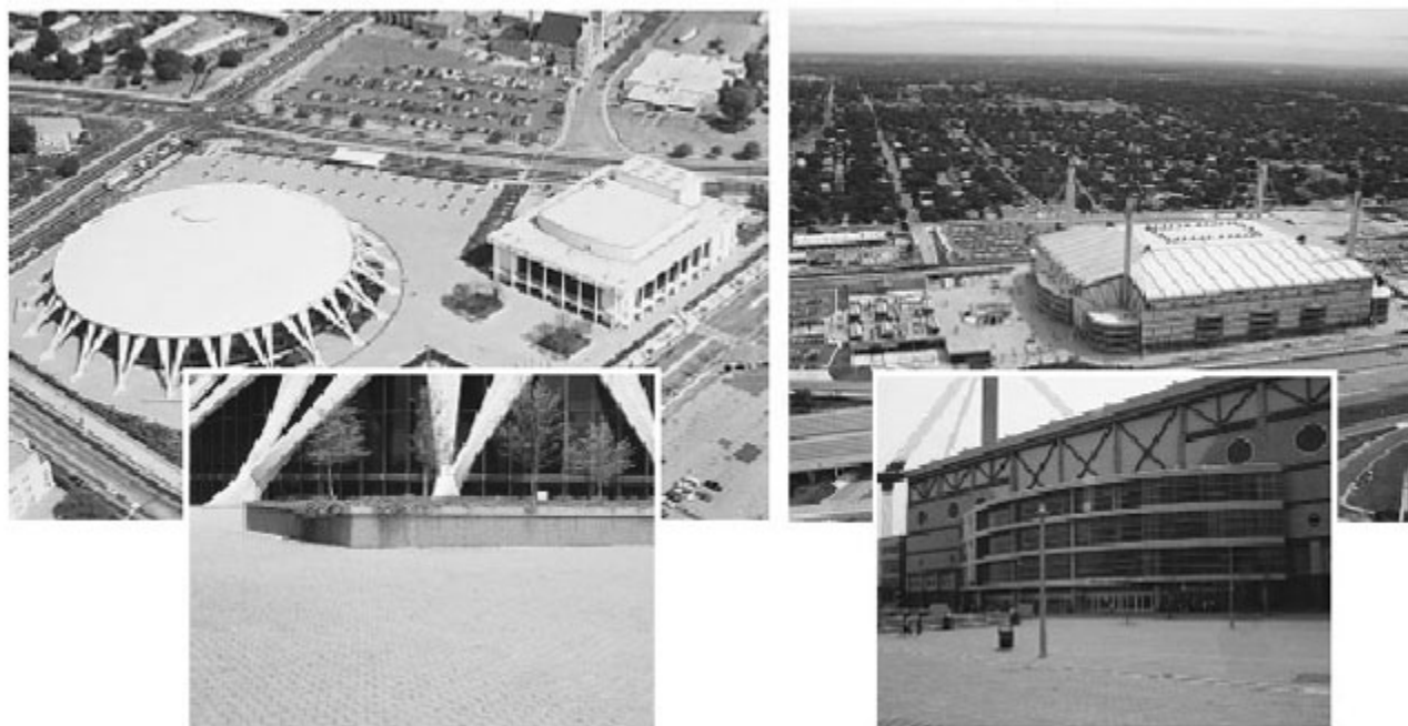
Figure 21. The plaza area around Scope Center in Norfolk, Virginia, (left) and one side of the Alamo Dome (right) in San Antonio, Texas, include roof plaza decks surfaced with concrete pavers.
