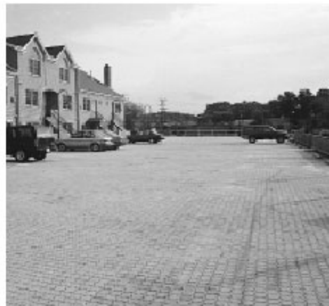
Figure 2. Concrete pavers serve vehicular traffic and parking over a concrete parking structure next to a residential development.
