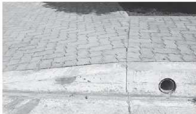
Figure 3. Ramp pavers changing angle.
