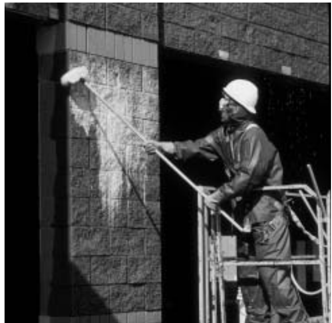
Figure 1 — Pressure Chemical Cleaning (photo courtesy of PROSOCO, Inc.)
